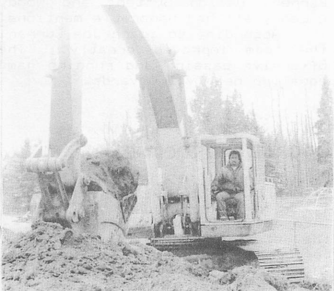
Work began on the library foundation during Homecoming week.
